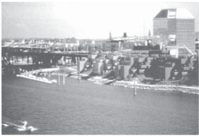
Fig. 24. 303 housing units at McCormick Pier.
